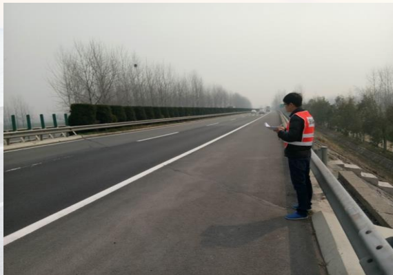
现场调查裂缝 field survey
