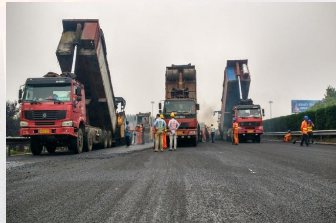
加宽段3台摊铺机 3 pavers for the regular section
