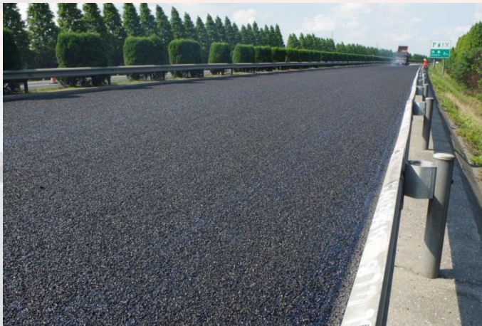
橡胶沥青碎石封层 Rubber modified bitumen chip seal
