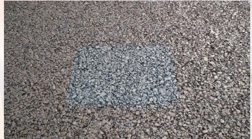
改性乳化沥青洒布后 after bonding layer laying
