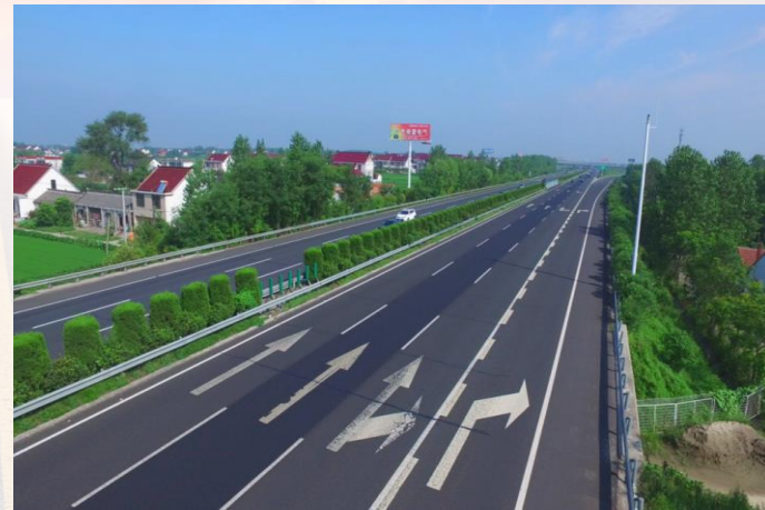
雾封层洒布后 after fog seal
