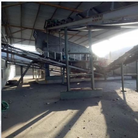
排水路面铣刨料破碎 crushing of milled porous asphalt
