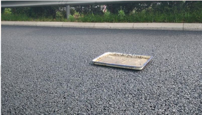
改性乳化沥青洒布前 Before bonding layer laying
