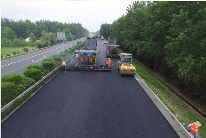
正常路段2台摊铺机 2 pavers for the regular section
