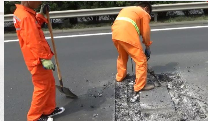
开挖观察裂缝 excavation for crack inspection
