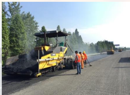
分车道摊铺 paving by lanes
