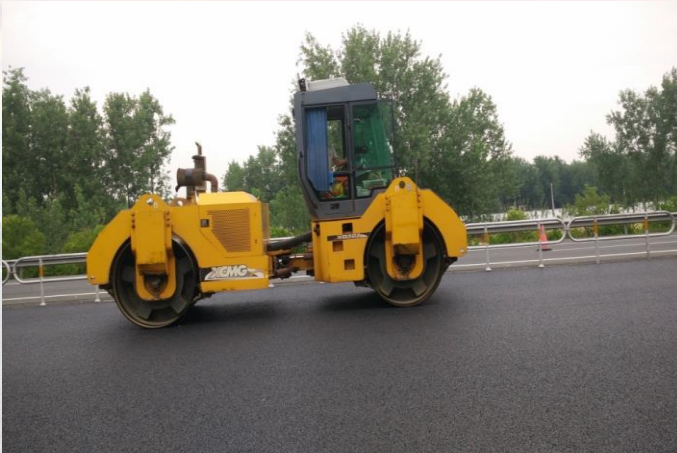
钢轮碾压 steel wheels compaction
