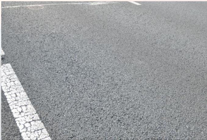
雾封层洒布前 before fog seal
