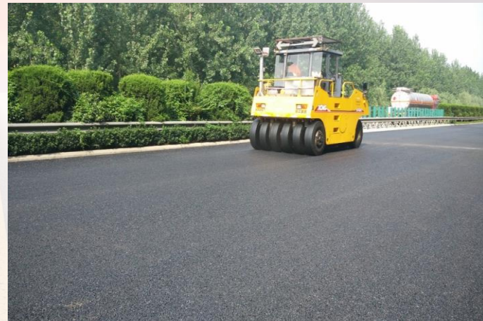
胶轮碾压 rubber tire compaction
