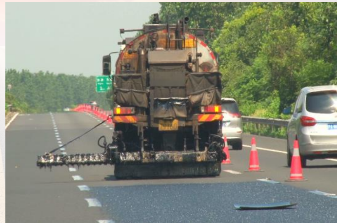
雾封层洒布 fog seal laying
