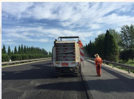
铣刨形成接缝 joint via milling
