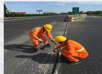
渗透性树脂涂抹 diffusible resin application
